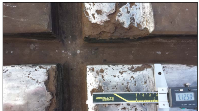
Figure 4. High Angle Crossing Diamond Flangeway Corner Impact Load Affected Zone (0.5-inch Wheel Drop)
