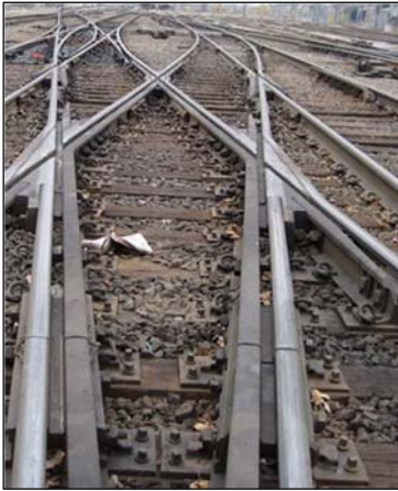
Figure 3. Switch Layout in a Passenger Yard
