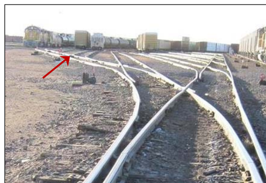
Figure 2. Switch Layout in a Freight Yard
