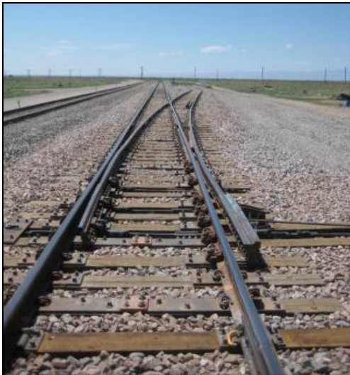
Figure 9. Prototype Continuous Rail Turnout at FAST
