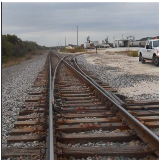
Figure 1. Prototype Continuous Mainline Rail Turnout in Service near Clifton, TX
