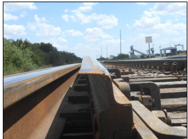
Figure 3. Left (Gage Side) Switch Point (End View)
