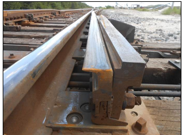
Figure 2. Right (Field Side) Switch Point (End View)
