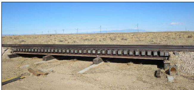
Figure 1. BDTF – Adjustable Three-Span Trestle for Evaluation of Onboard Bridge Deflection System
