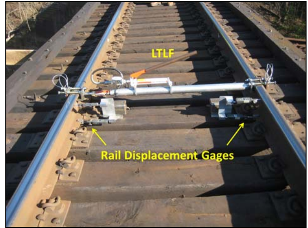
Figure 4. LTLF applying Gage Spreading Forces to the Railhead
