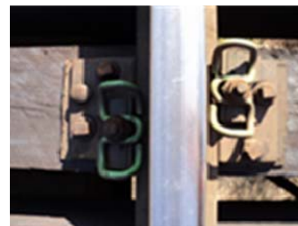
Figure 2. Vossloh 16-inch Rolled Plate BTE-30 System
