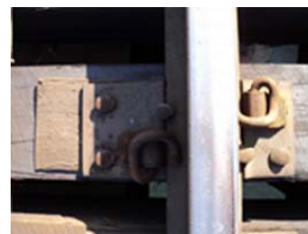
Figure 3. Pandrol 18-inch Rolled Plate Victor System
