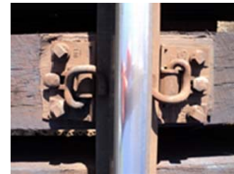
Figure 1. Pandrol 16-inch Cast Plate System
