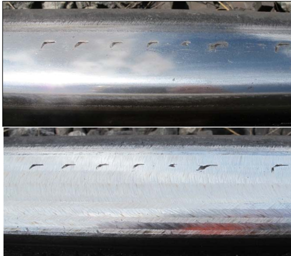
Figure 3. RCF markings on top of high rail at 300 MGT of accumulated tonnage in the IS rail curve. Top image shows rail before grinding and bottom image indicates rail after grinding.
