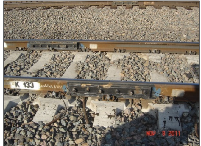
Figure 6. HFTs supporting a Pair of IJs at a Control Point
