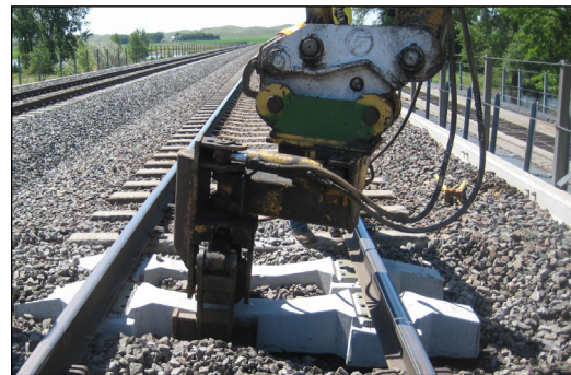
Figure 2. Installation of the HFTs on the Bridge Approach
