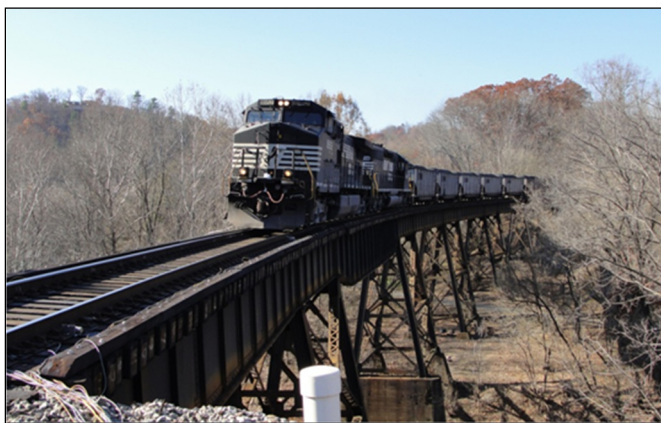
Figure 1. Test Bridge over the Roanoke River at MP V257.5
