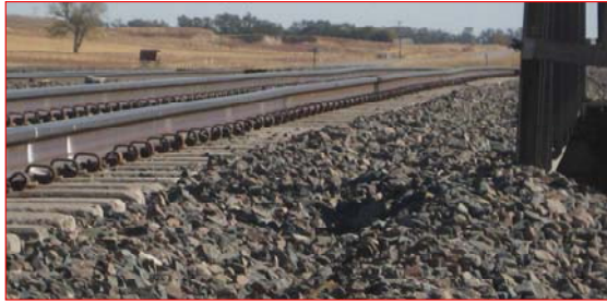
MP 78.2, two years (480 MGT) after ballast mat/drainage installation
