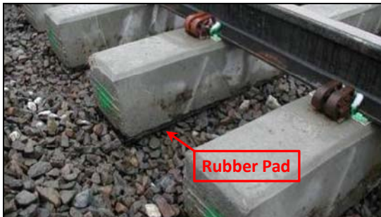
Figure 3. Concrete Ties Fitted With Rubber Pads
