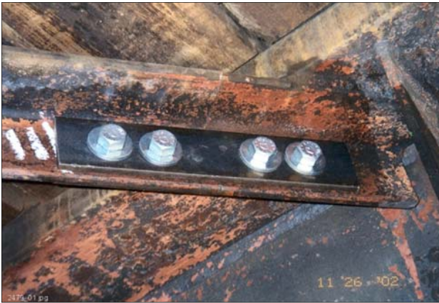
Figure 3: Simple Bolted Splice Repair to Top Lateral Brace
