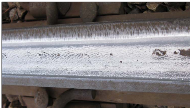
Figure 4. Low Rail at Wabun, Virginia, prior to Grinding
