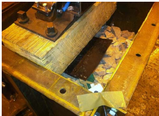
Figure 4. Detail of MBTSS/Protection beneath Tie
