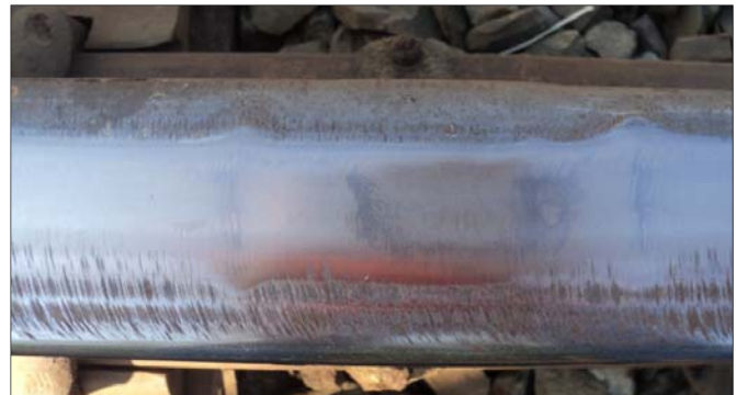
Figure 5. Untreated Thermite Weld Running Surface at approximately 36 MGT, 5 MGT after Rail Grind
