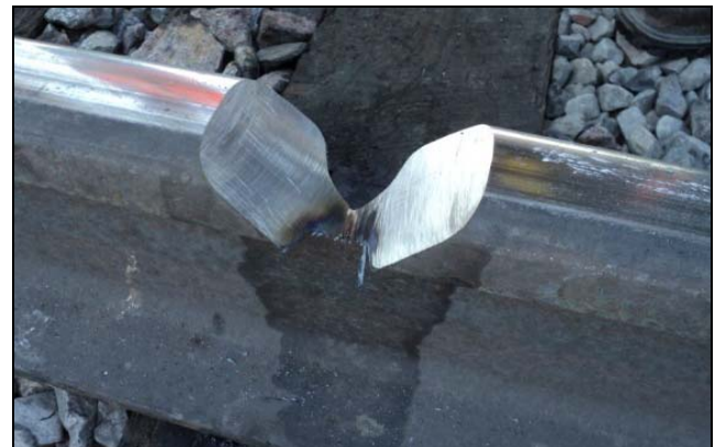
Figure 2. V-cut made in Railhead using Rail Saw and Angle Jig
