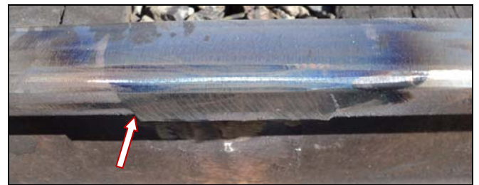
Figure 8. HDR Weld after Production (Arrow indicates geometry transition at the bottom of the railhead that acted as a stress concentrator)
