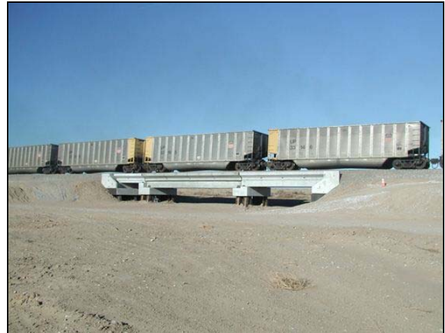
Figure 2. SOA Concrete Bridge at FAST
