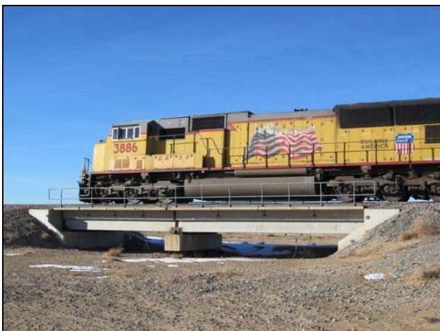
Figure 1. Conventional Concrete Bridge at FAST
