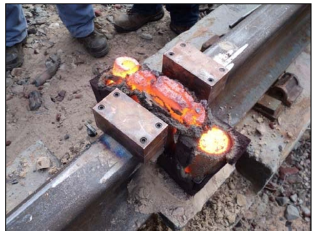
Figure 3. Two Chill Blocks placed adjacent to Sheared Head Material. Chills are applied Immediately after Shearing
