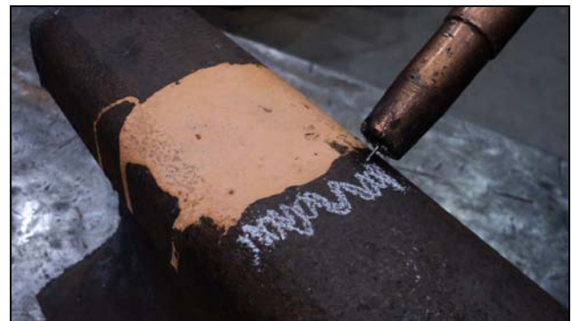
Figure 5. Mockup Showing Application of Surface Hardening Material over HAZ next to Weld (Orange paint represents sheared head riser, and white chalk marking indicates location of applied hardening material)
