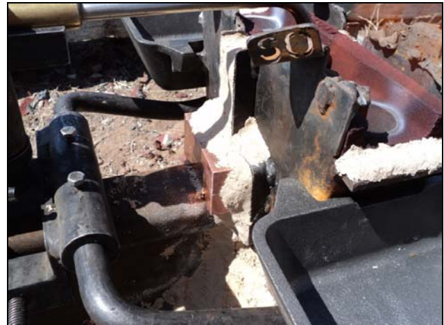
Figure 2. Single Chill Block Placed Flush to Weld Mold and Packed with Luting Sand. Chill is Applied throughout Weld Preheat and Pour
