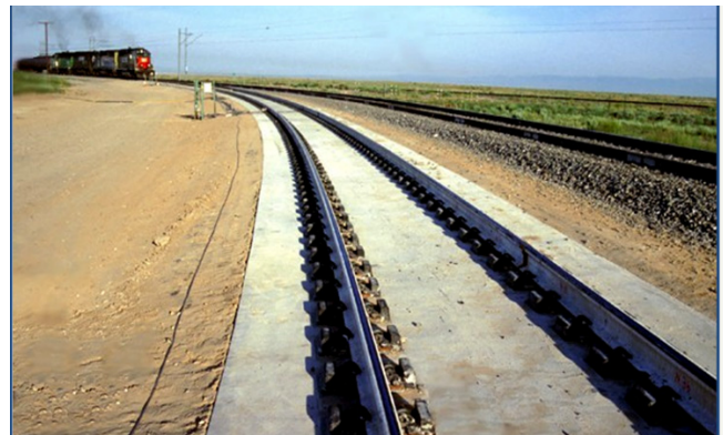
Figure 1. DFST Slab Track at FAST
