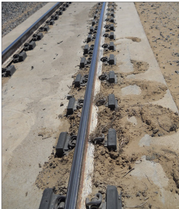
Figure 4. Direct Fixation Slab Track
