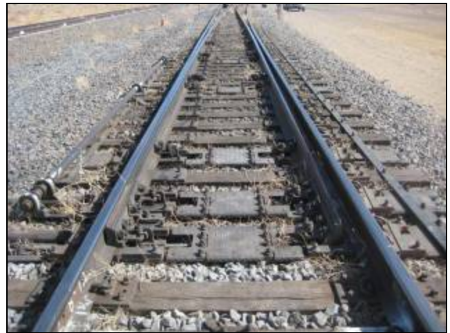
Figure 2. Conventional Split Switch Turnout at FAST
