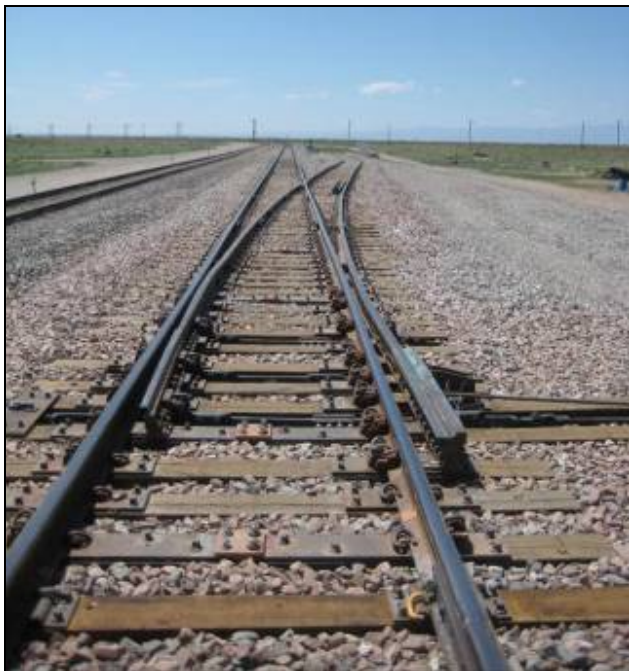
Figure 1. Prototype Continuous Rail Turnout at FAST
