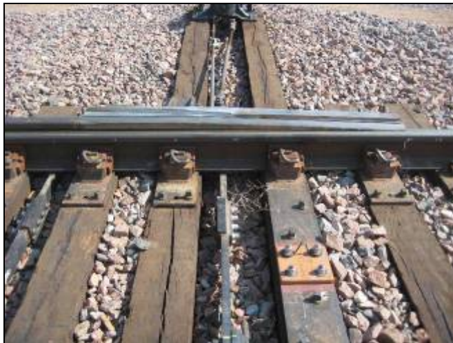
Figure 3. Vertical Ramping in Prototype Switch Points
