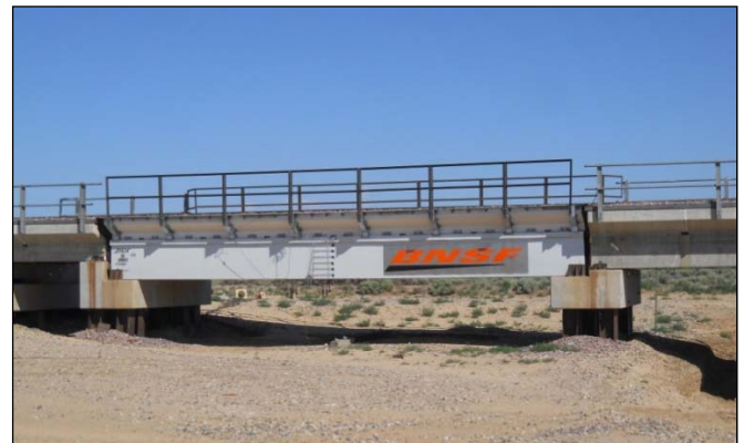
Figure 2. 42-foot HCB Span installed at FAST
