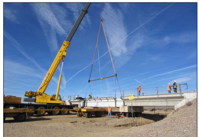
Figure 3. Removal of 42-foot Span at FAST
