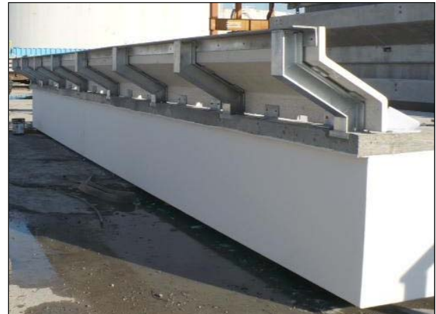
Figure 1. View showing Polymer Concrete Ballast Curb Panels and Steel Supports
