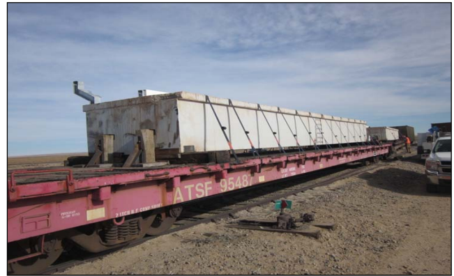
Figure 8. 42-foot HCB Span Ready to be Moved
