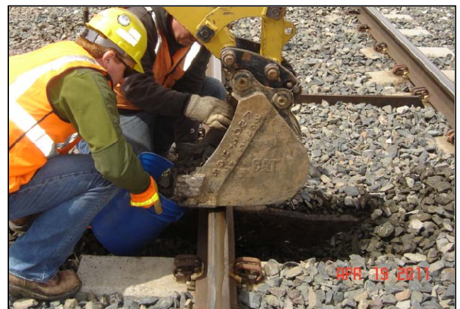
Figure 2. Ballast Sampling with Backhoe
