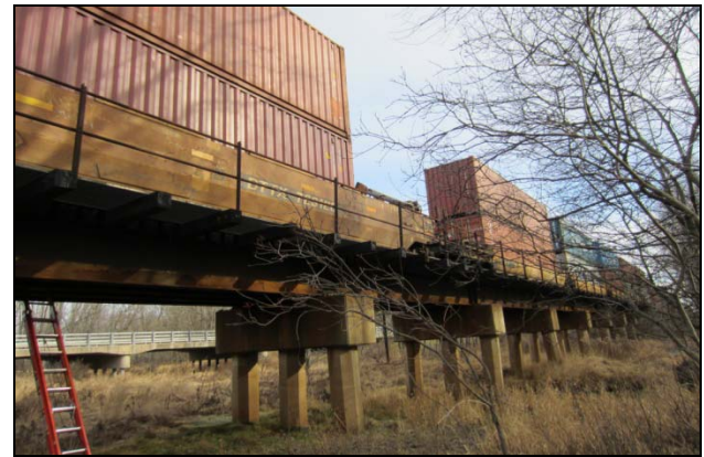
Figure 1. CN Test Bridge near Stevens Point
