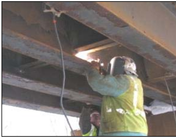
Figure 7. Welder Repairing Cracked Detail
