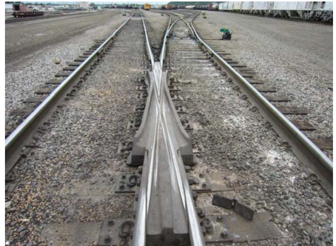
Figure 2. Self-Guarded Solid Manganese Frog In Revenue Service
