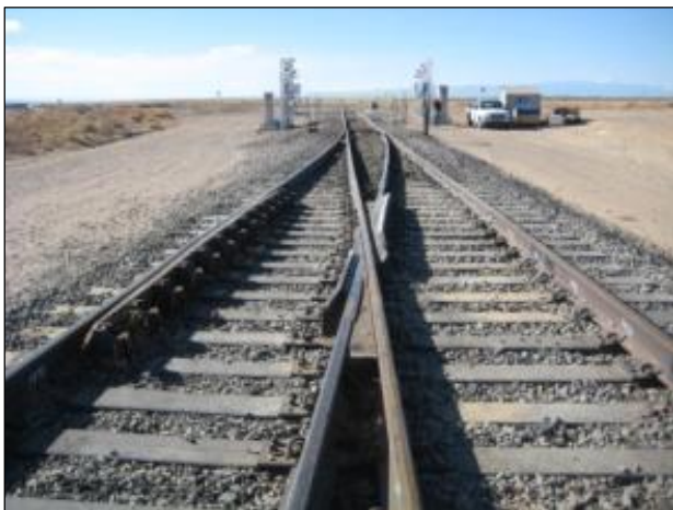
Figure 1. Lift Frog in High Tonnage Loop at FAST
