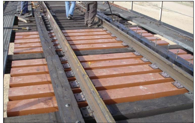
Figure 1. Bridge Deck Tie Tests on Vintage Span
