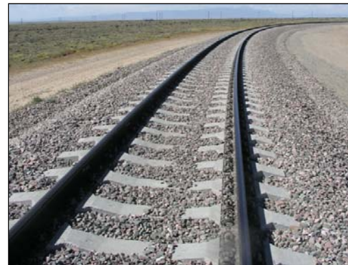
Figure 4. Improved Strength Track with Half-Frame Ties
