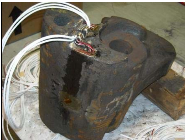
Figure 4. Strain Gages Installed
