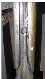
Figure 5. Switch Point with a 1/8-inch Gap
