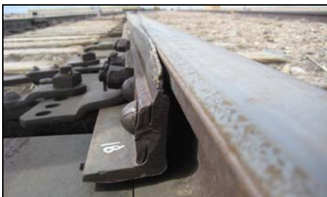
Figure 5. Switch Point with a 1/8-inch Gap
