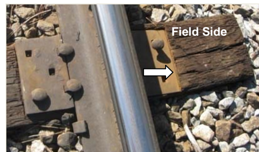
Figure 8. Tie Plate Cutting
