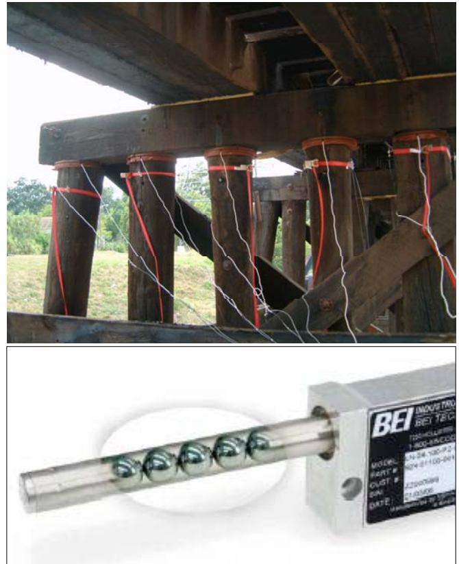
Figure 2. Timber Bridge Pile Capacity Field Assessment
