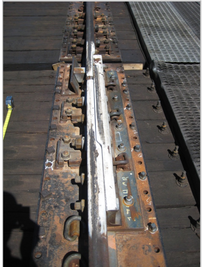
Figure 1. Rail Joint Detail for One Running Rail
