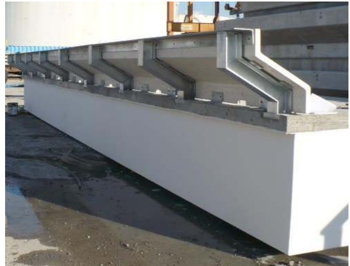
Figure 2: View Showing Polymer Concrete Ballast Curb Panels and Steel Supports
