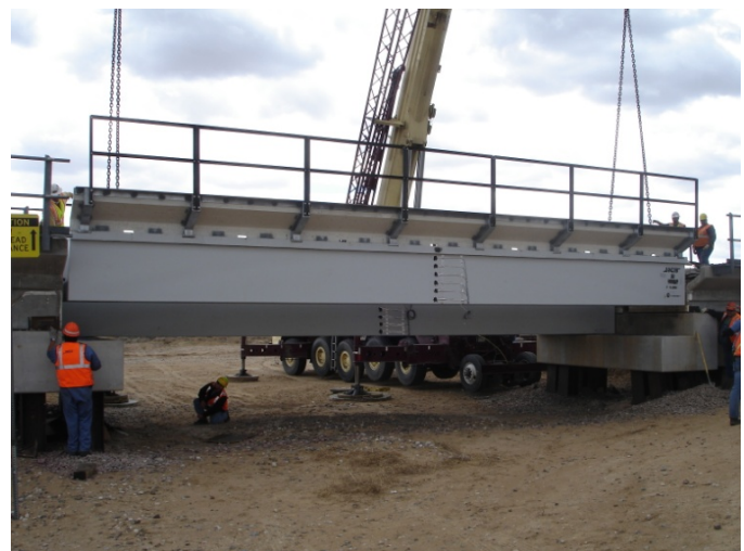
Figure 3. Installation of 42-foot Span at FAST
