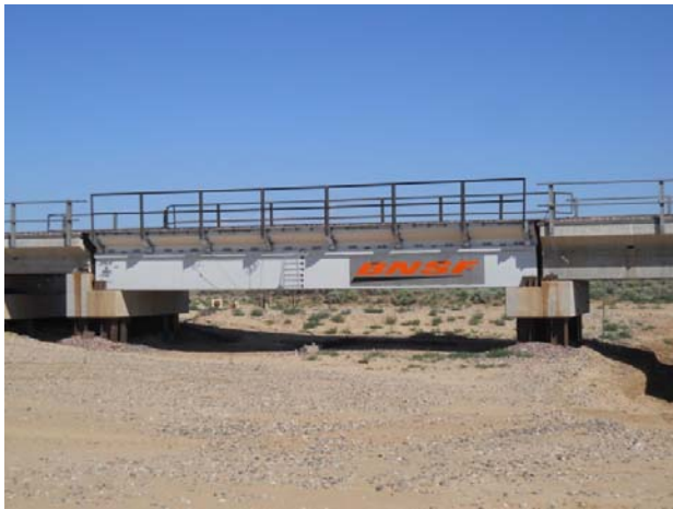
Figure 4. Completed Installation of 42-foot Span at FAST
