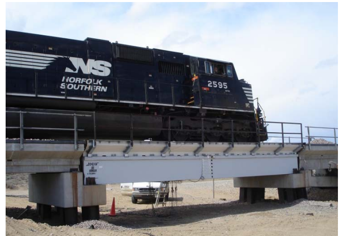
Figure 6. Train at FAST Passing over HCB Span at FAST
