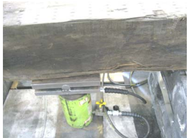
Figure 11. SYP 2 – Failure at Bottom Surface of Tie
