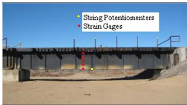
Figure 5. Vintage Riveted Span at FAST
