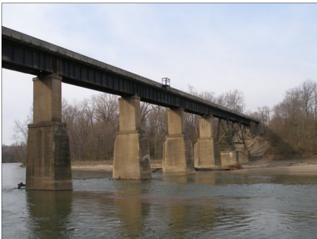
Figure 1. Vintage Riveted Steel Span in Revenue Service on NS
