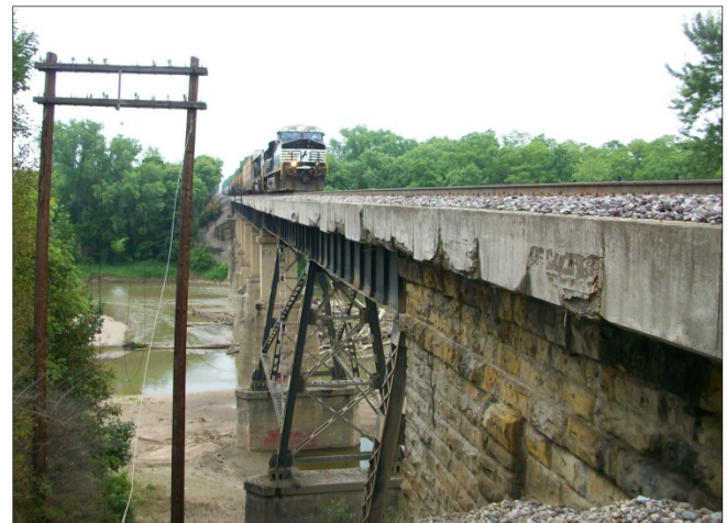
Figure 3. 1912 Vintage Riveted Span with Ballasted Deck on NS
