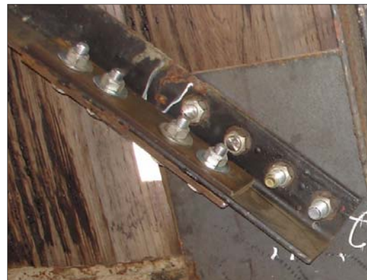
Figure 5. Splice Repair to Vertical Leg of Top Lateral Brace
