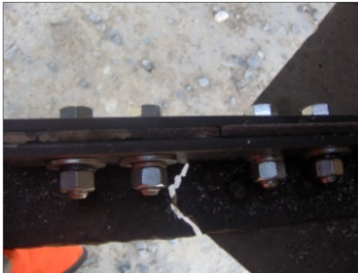
Figure 3b. Splice Repair
