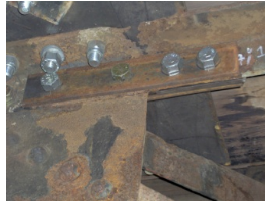
Figure 4b. Splice Repair to Vertical Leg of Cross Frame Member
