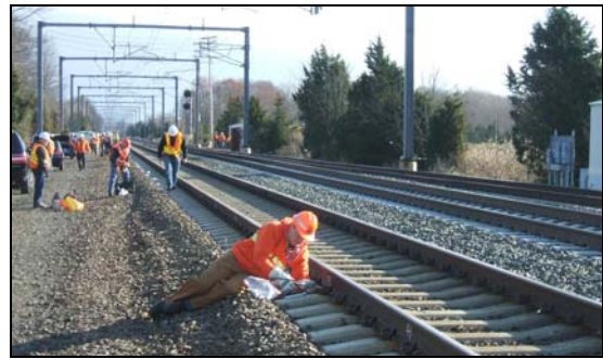
Figure 3. Amtrak Field Site near Guilford during Installation of Test Connections
