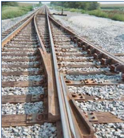
Figure 5. Partial FB Turnout Frog (Lift Frog)
