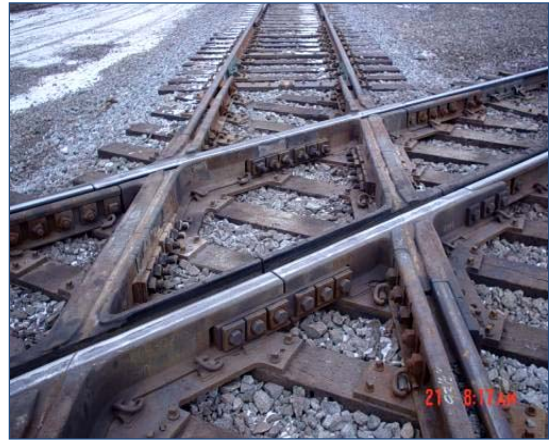
Figure 2. OWLS Flange Bearing Crossing Diamond
