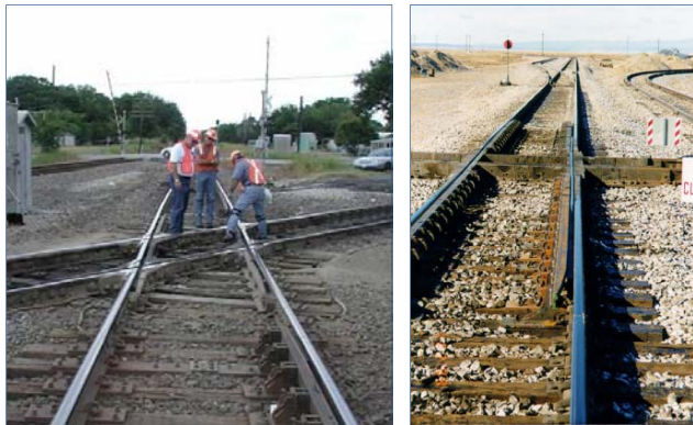
Figure 1. Tread Bearing (Left) and Flange Bearing Crossing Diamonds
