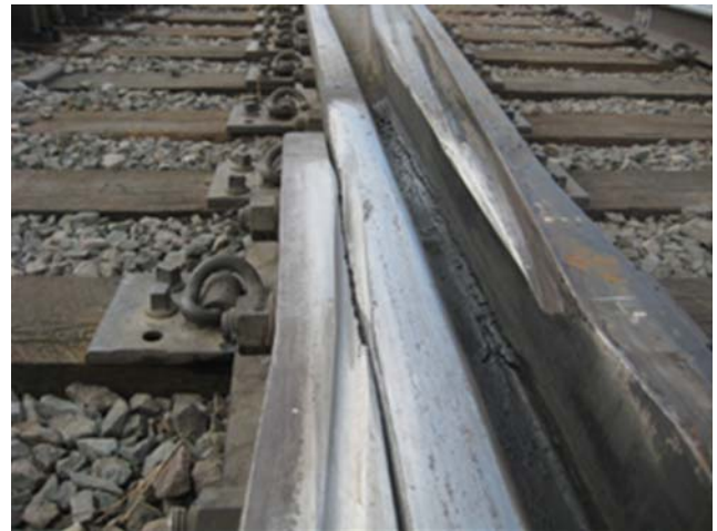
Figure 4. Cross Grooving in Flange Bearing Turnout Frog
