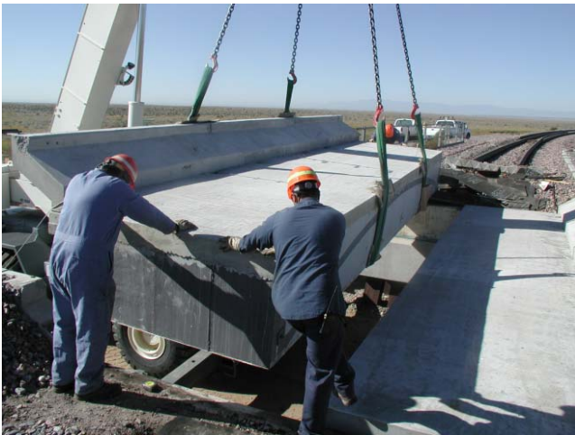
Figure 3. Installation of HCB Span with New Deck at FAST
