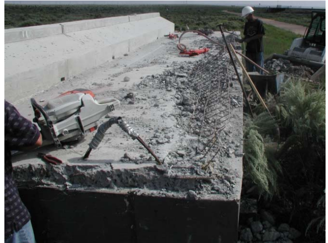
Figure 4. Removal of 4-inch Concrete Deck
