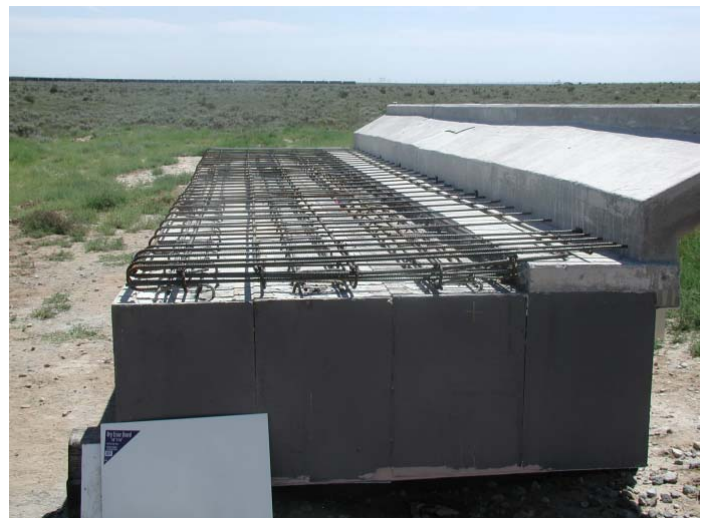
Figure 5. Reinforcement for New 6-inch Deck
