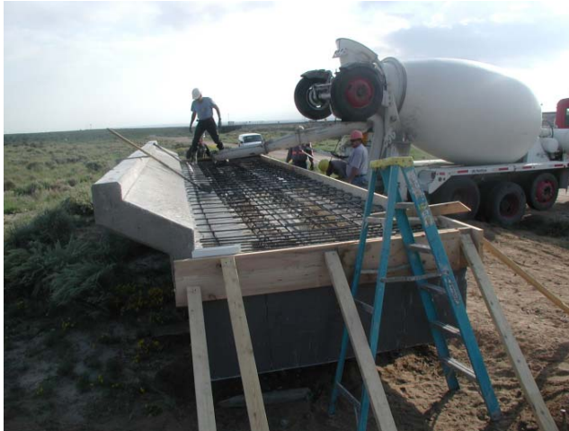
Figure 6. Concrete Pour for New Thicker Deck
