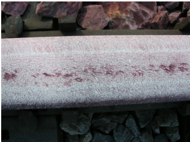
Figure 8. Low Rail of Curve S in the TOR-treated Zone at Site 3 End of Test June 2009
