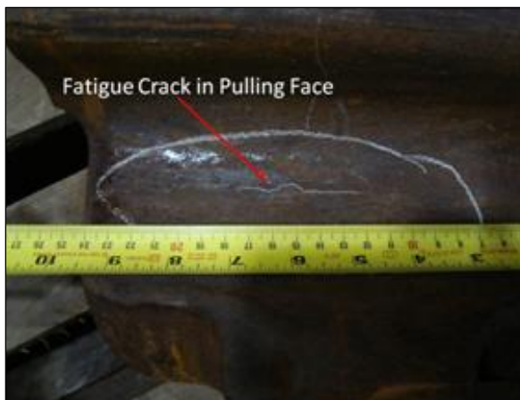
Figure 1. Fatigue Crack on the Pulling Face of a Knuckle
