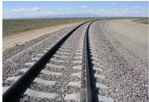
Figure 3. Improved Strength Track with Heavy-Duty Ties
