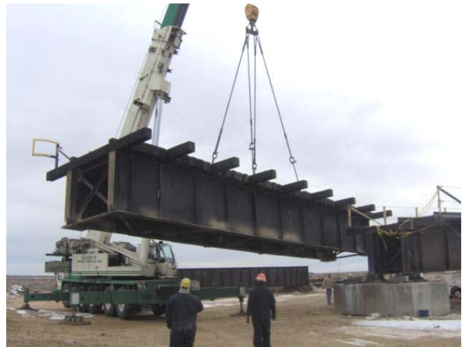
Figure 2. 1912 Riveted Steel Span being installed at FAST
