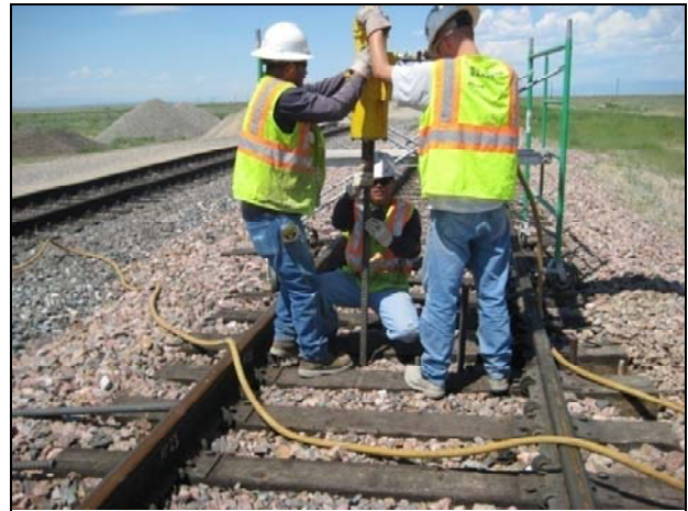
Figure 6. Installation of the Minipiles at the FAST
