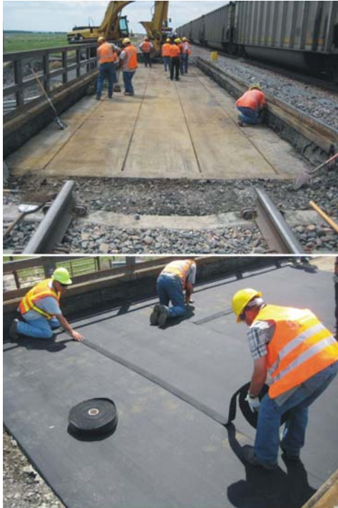
Figure 2. Ballast Mats for a Bridge at Western Mega Site
