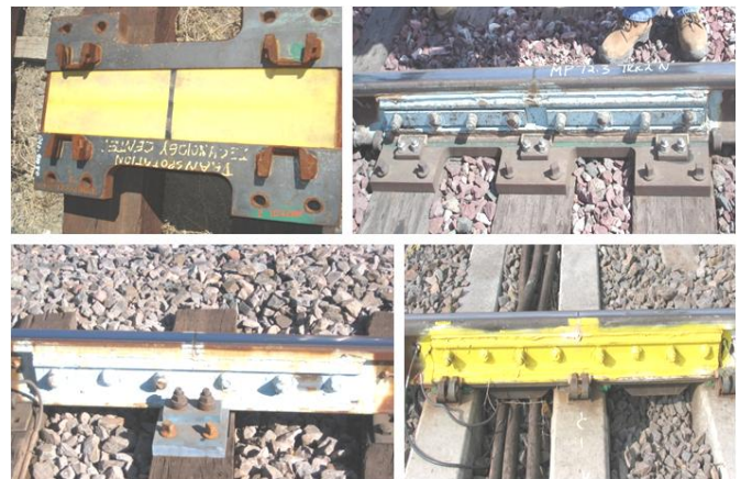
Figure 5. Clockwise from top left corner: Two-Tie-Plate, Three-Tie-Plate for Timber Ties, Three-Tie-Plate for Concrete Ties, and Single Tie Plate
