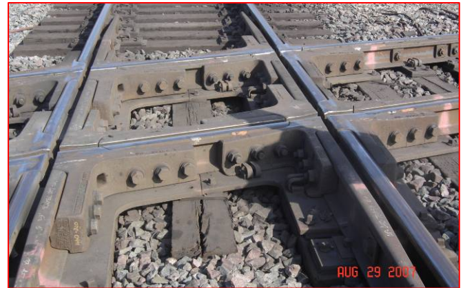
Figure 2. Diamond Crossing Installed in 2007 (looking east)
