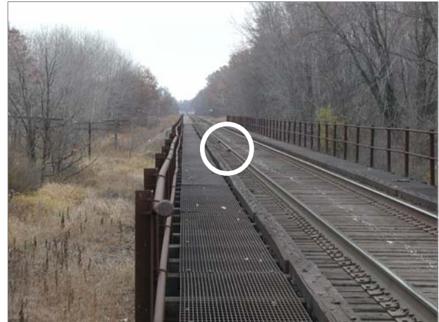
Figure 5: Bolted Rail Joints on East Rail above Span 5 and Span 6
