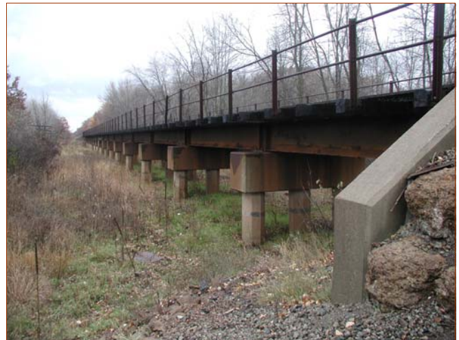
Figure 2: Overview of Test Bridge
