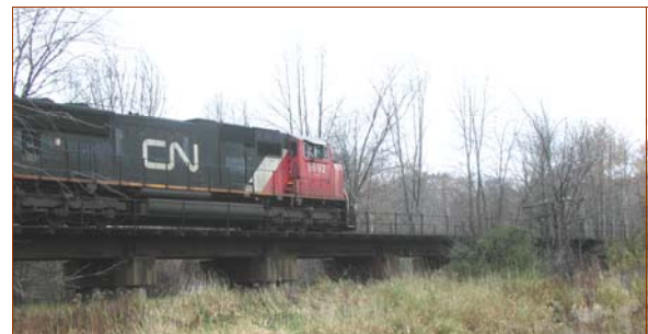
Figure 11: Train on Test Bridge
