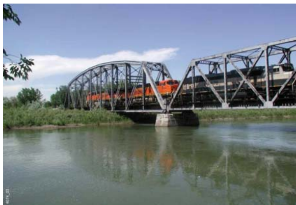
Figure 2. BNSF 400-foot Steel Bridge
