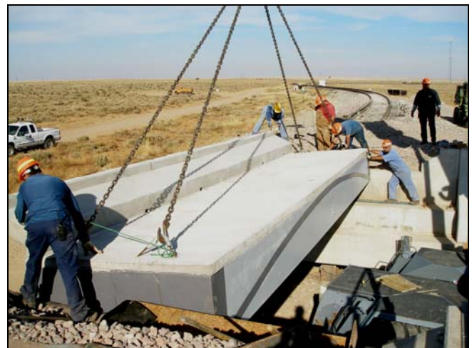
Figure 2. Installation of HCB Prototype Span at FAST
