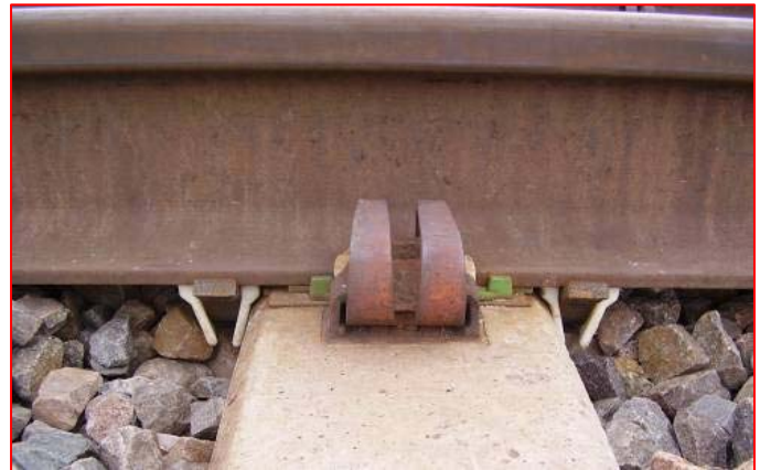
Figure 2. Box Anchors of Rail at Test Site
