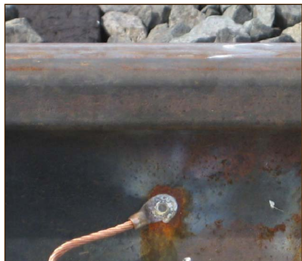
Figure 2. Pin-Brazed RWI
