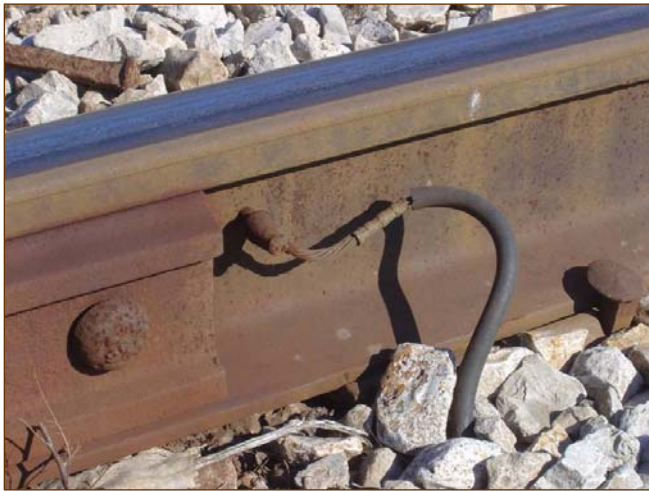
Figure 3. Tapered Pin RWI (i.e., Chicken Head)
