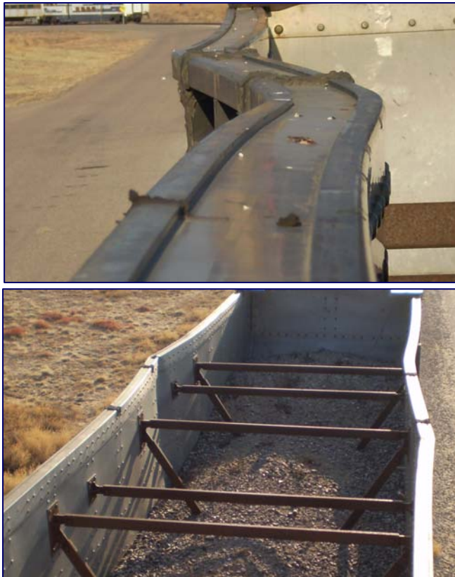
Figure 3. Buckled Top Chords
